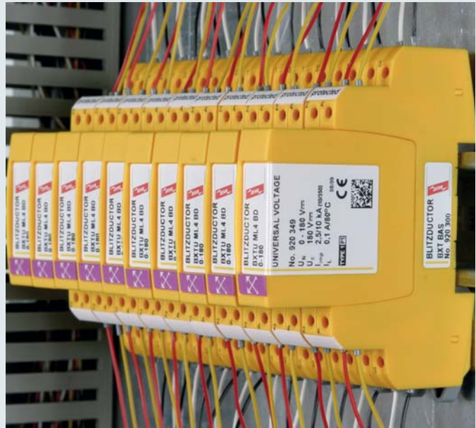
Example of use of BLITZDUCTOR XTU.
